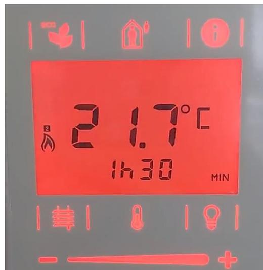
Figure 8: Time-to-setpoint implementation on the room thermostats. The thermostat shows indoor air temperature and the time-to-setpoint estimate.
