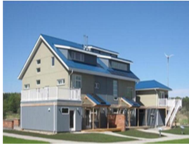
Figure 3: South-West view of House A and House B
