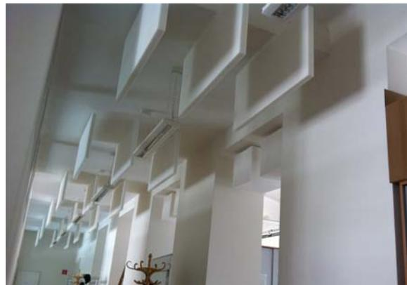
Figure 5 Added absorption elements in OP
