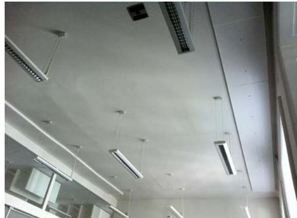
Figure 4 Added absorption elements in SR
