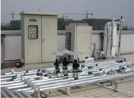
Figure 10. Demonstration hybrid HP system
