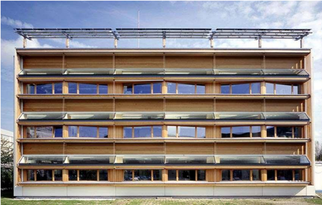
Fig. 15 – Picture of the LE South façade (credits: CHABOD Louis, 21.10.2012)
