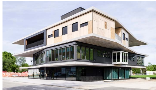
Figure 1: The NEST building (Empa, 2016).
