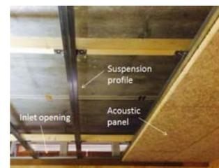
Figure 3 Diffuse ceiling setup
