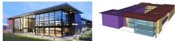
*Figure 1: NIMBUS building and its EnergyPlus model*
