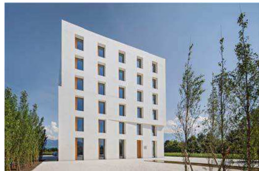
Figure 1 The “Concept 2226” building in 2014 (Photo: E.Hoeber)
