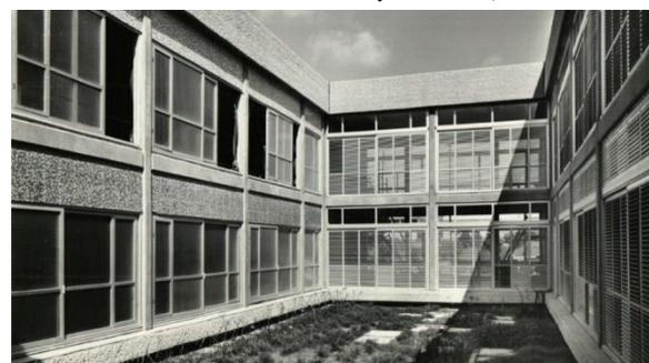
*Figure 6: Gilman Building, the smaller courtyard of the southern wing, looking east, ca. 1966 (courtesy of Israel Stein). The corridor facades, here facing north and west, were screened with sliding aluminium panels of rotatable PVC slats*
