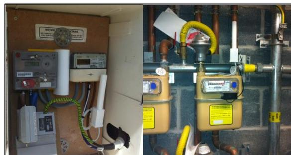
Figure 4 Pulse output sensors connected to the electricity meter (left) and gas meter (right)
