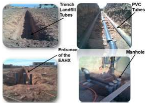
Figure 2: Implementation details of the EAHX.
