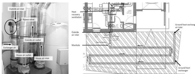
Figure 3. Details of the exchanger network
