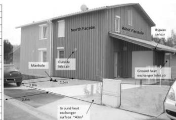
Figure 1. House and ground heat exchanger data
