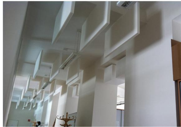
Figure 6 Added absorption elements in OP
