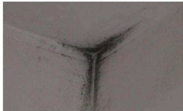
Figure 1. Mould growth at the upper corner surface.
