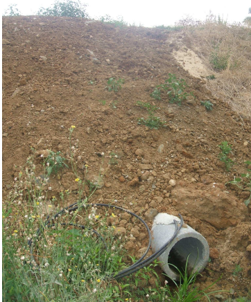
Figure 2: Showing the outdoor entrance of the buried pipes
