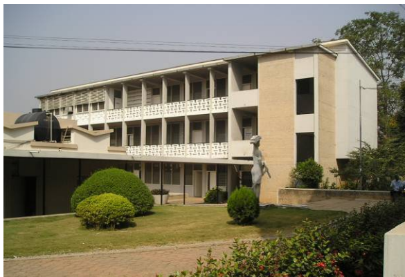
Figure 2 External view of building CAP
