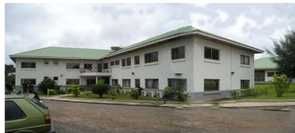
Figure 4 External view of building KCR
