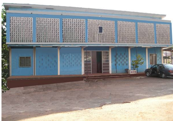
Figure 10 External view of building DCD
