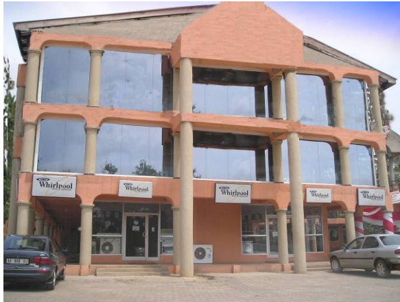
Figure 8 External view of building ROY
