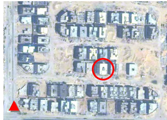
Figure 1.a: 0.6m resolution Quick bird 2008 satellite image of the site and building examined in the study.
