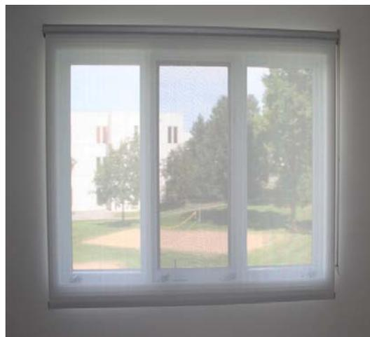
Figure 2 Close-up picture of the interior reflective and perforated screen shades installed on the windows of the Test House
