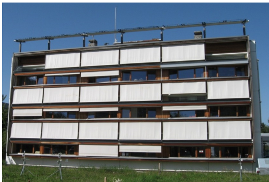
Figure 1 General view of the LESO building
