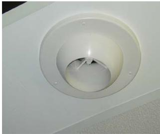
Figure 1b Nozzle diffuser
