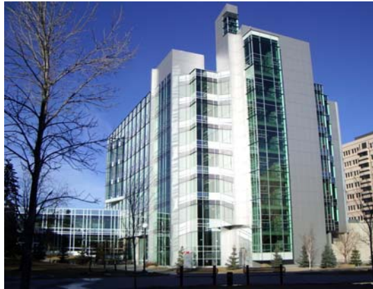
Figure 1 Perspective view of ICT Building from southwest
