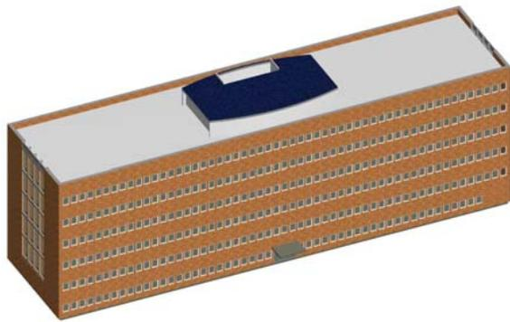
Figure 1. View of the glazed reference building, where the glazed area is 30 % of the façade area.
