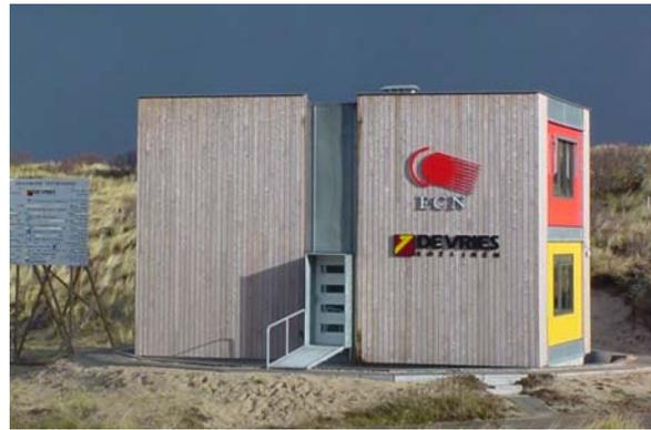
Figure 4 Research facility containing four rooms each holding a different façade. The bottom room on the right contains the parallel window; the bottom room on the left contains the panels.
