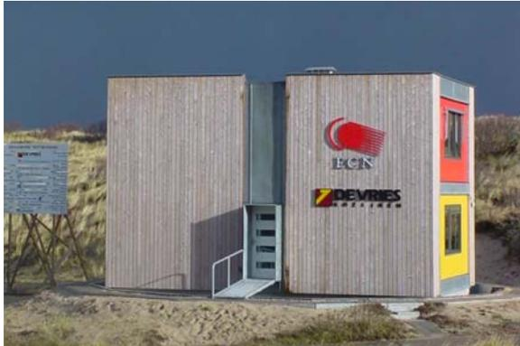
Figure 1 ECN research facility containing 4 separate rooms each holding a different façade.
