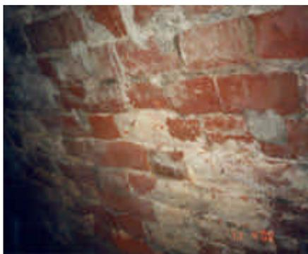
Figure 3 Efflorescence and crypto-efflorescence damages on the vault ceiling
