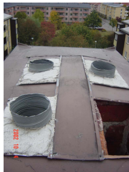
Figure 15. Exhaust ducts for relative humidity measurement
