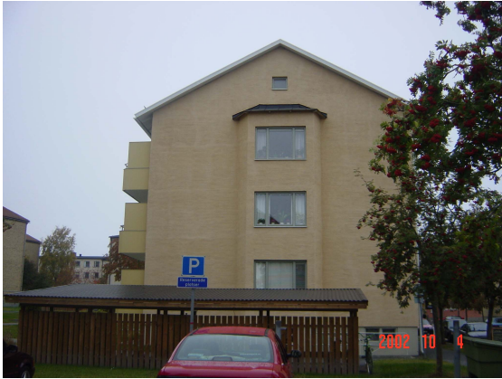
Figure 14. An experimental multi-family house in Gävle
