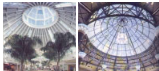
Figure 1. The West Oak Mall (U.S.A.) and the Iguatemi Shopping Center, Brazil: similar architectural solutions for different climatic contexts (Source: AMORIM, 2001).
