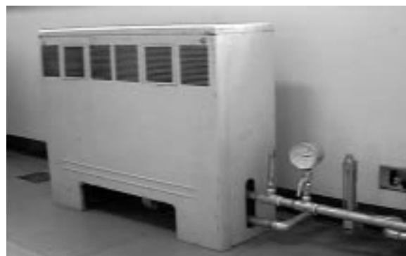
Fig.1 Cabinet convector with three row finned-tube heating elements in reference room (heating performance 790 \text{ Wm}^{-2} under design conditions: steam temperature 375 K; inlet air temperature 291.5 K).
