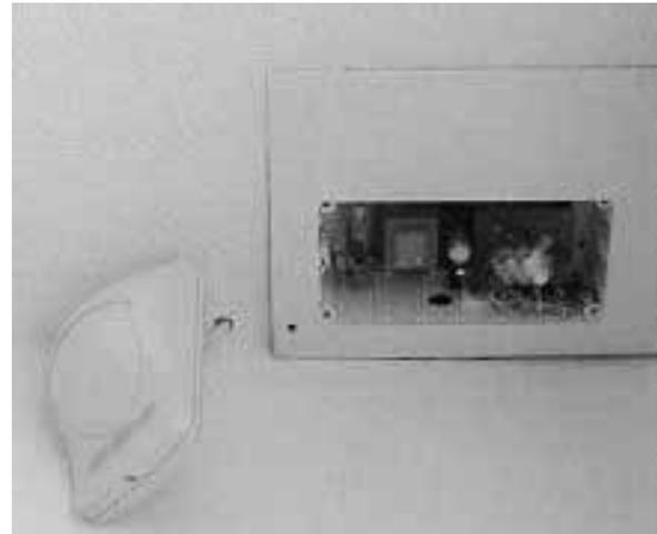
Figure 2 *Roomcontroller and PIR detector*
