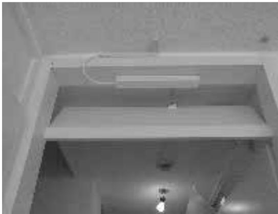
Figure 4: Automatically opened passage between living room and corridor for natural based ventilating system
