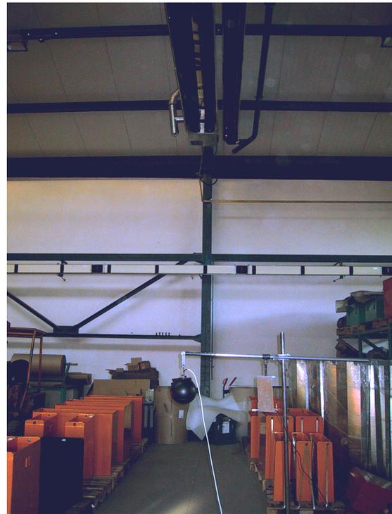
*Fig.1 Example of the industrial hall heated by IR radiant heating*
