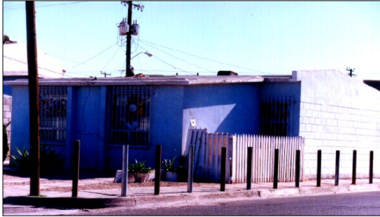
Photo 2.- Mexicali housing: concrete roof and concrete block walls
