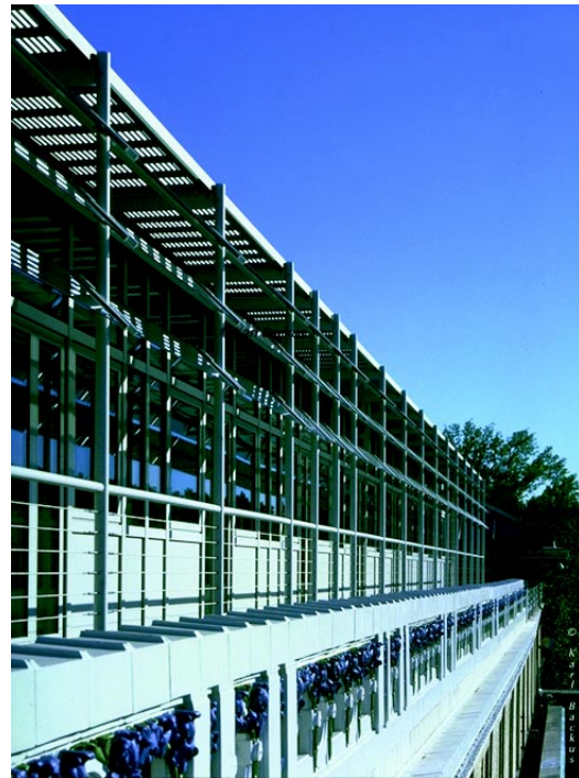
FIGURE 10. Exterior view of the Robert L. Preger Intelligent Workplace at Carnegie Mellon University. The IW incorporates dynamic enclosures and task-ambient HVAC systems to reduce energy needs.
